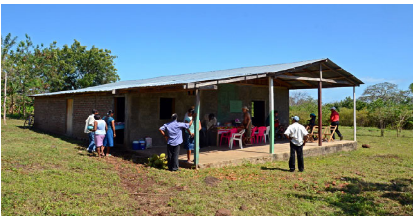
Productores Orgánicos de Ometepe, one of two cooperatives that sell coffee to the Sister Islands, completed its new beneficio, or coffee processing plant, in 2011. The plant is midway between the communities of La Palma and El Corozol, on the road past Balgüe.
