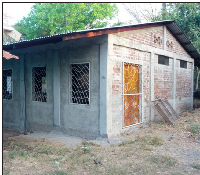
The future Tostadores processing facility at Mano Amigo
